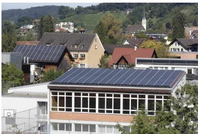
Photovoltaic panels on roofs in Zwischenwasser
